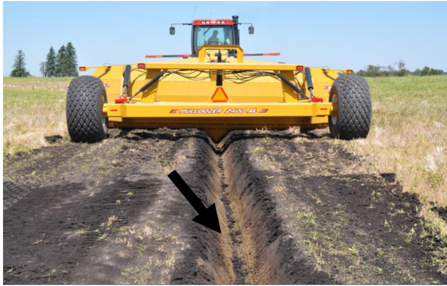
Figure: Trench after the operation with no wind row ridges of dirt left
