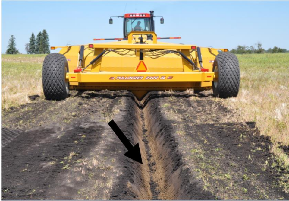
Figure 3: Trench after the operation with no wind row ridges of dirt left
